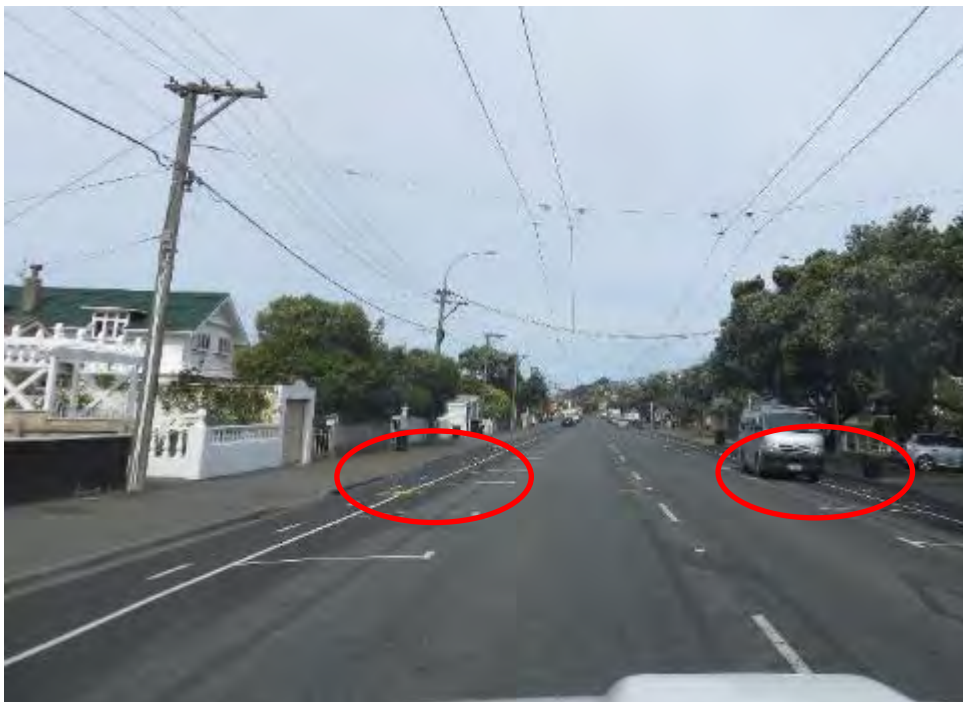
Figure 2-32: Photo showing a lack of no-parking line marking between larger parking spaces
