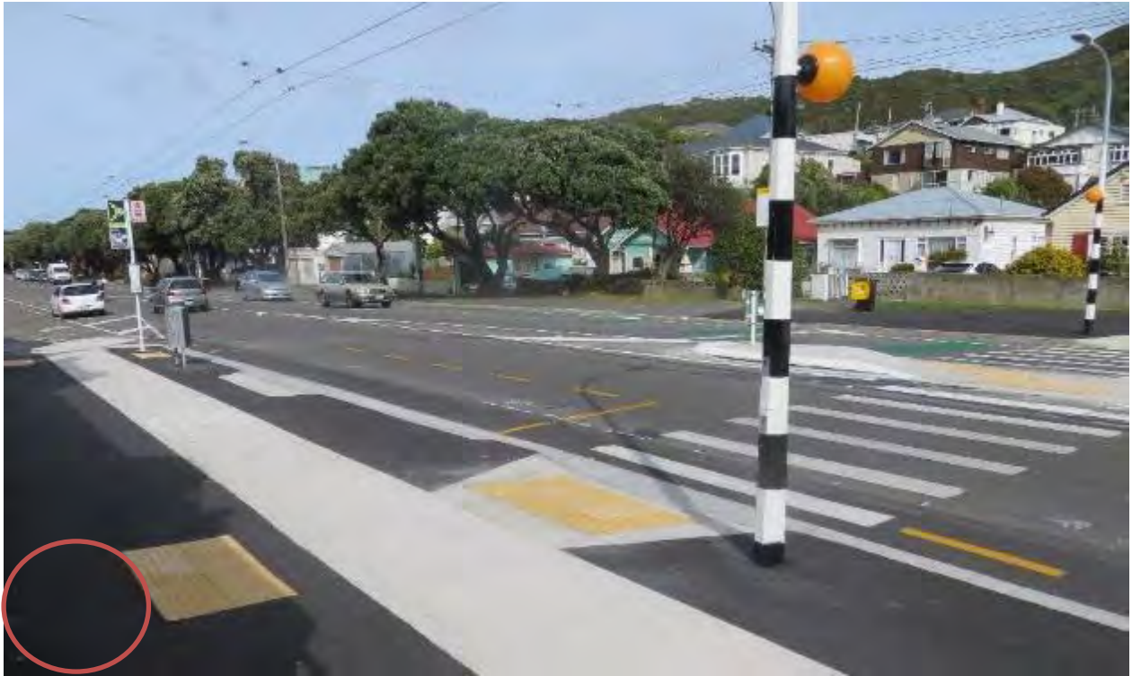
Figure 2-26: Photo showing missing directional tactile pavers on the eastern side of the pedestrian zebra crossing located south of Dee Street.
