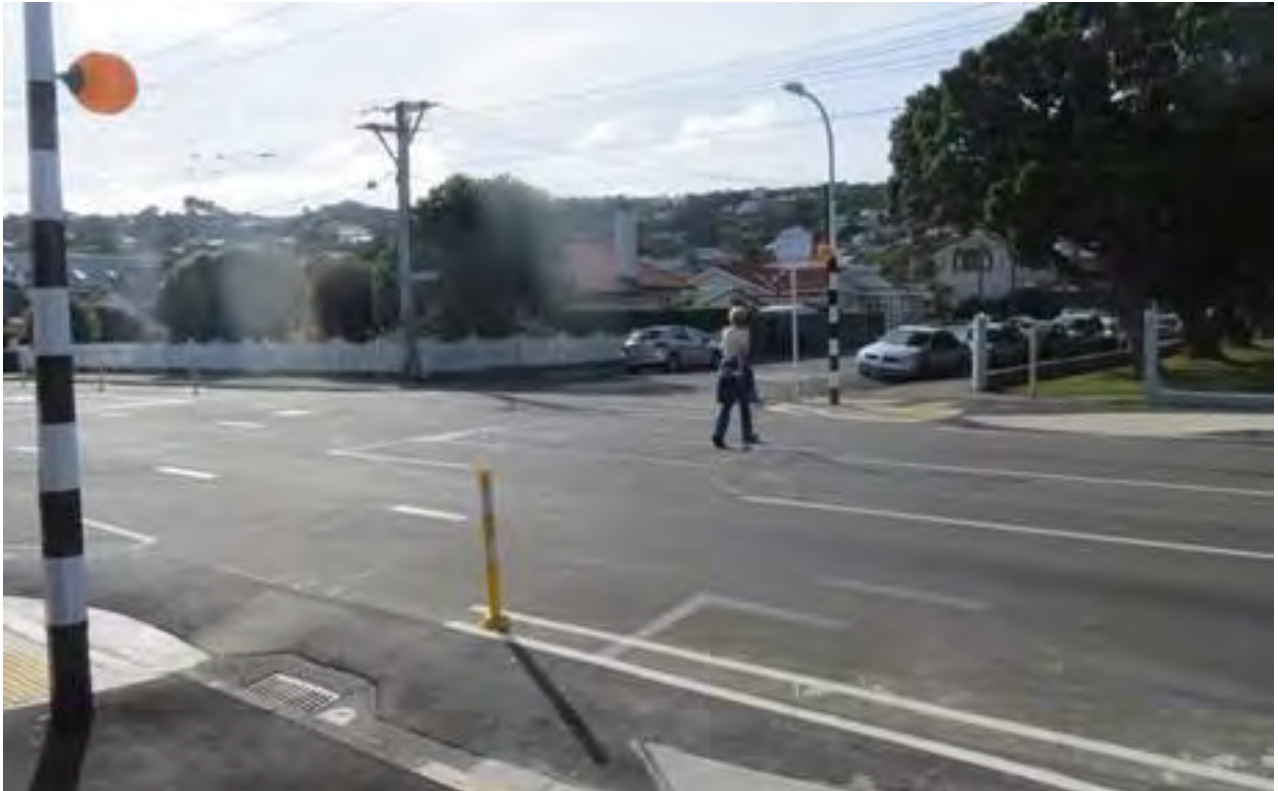
Figure 2-20: Photo showing the partially built pedestrian zebra crossing south of Humber St Recommendations
