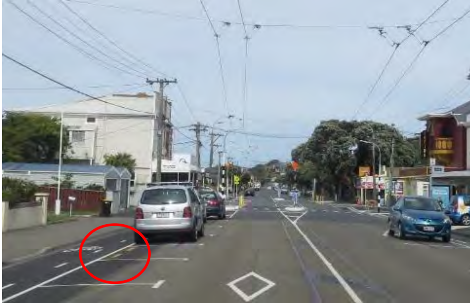
Figure 2-31: Photo showing no-parking line marking between parking spaces, north of Mersey St
