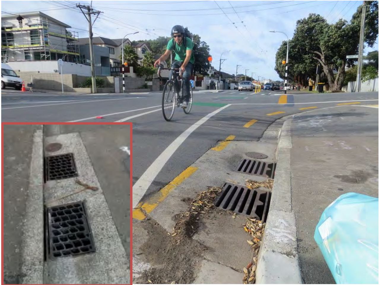
Figure 2-18: Photo showing a non-cycle friendly sump at Tamar St/The Parade (inset photo: example of cycle friendly sumps elsewhere along the route).
