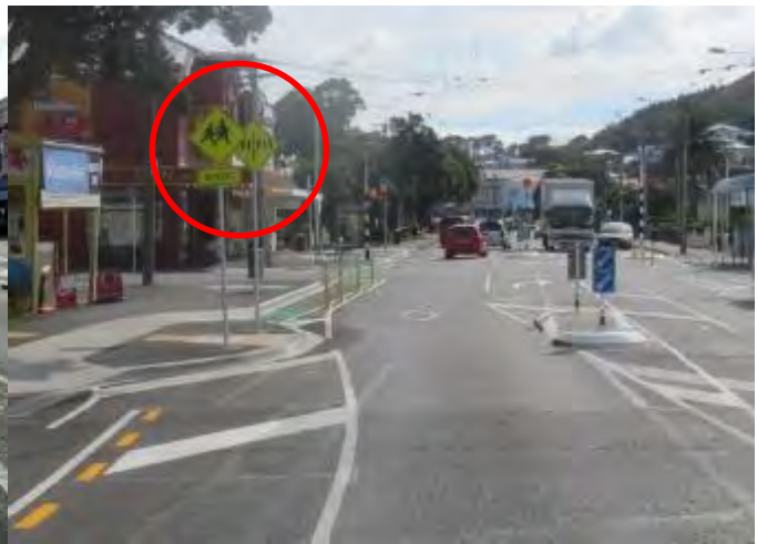
Figure 2-25: View northbound on The Parade approach to the pedestrian refuge island. Note the partially overlapping of the pedestrian crossing signage by the school sign
