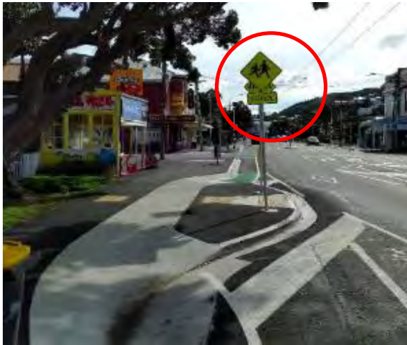
Figure 2-24: View northbound on cycleway approach to the bypass of the pedestrian refuge island. Note the overlapping school and pedestrian crossing signage south of Mersey Street.
