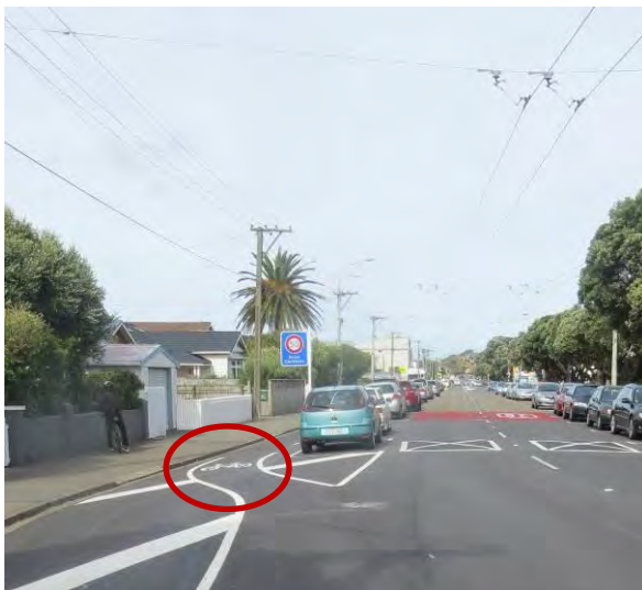
Figure 2-5: Photo showing a lack of green coloured cycleway markings on diverge from the "sharrow" lane into the cycleway
