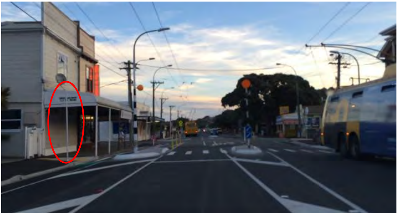
Figure 2-28: Photo showing a pole without a Belisha Beacon Disk or black and white markings on the pedestrian zebra crossing (eastern side) located north of Mersey Street.
