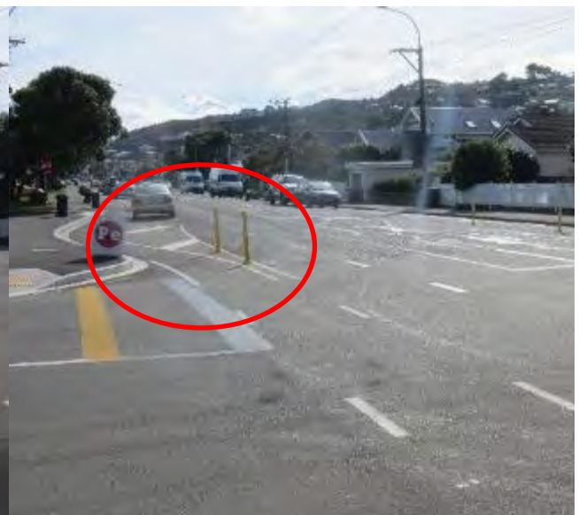
Figure 2-22: Photo showing the safe-hit posts installed at the western side of the Humber St intersection
