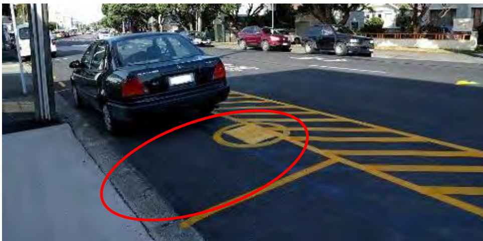
Figure 2-29: Photo showing the length of the southern disabled parking space (note the vehicle parked at the southern end of the space) and the fire hydrant located between the two parking spaces (currently located inside the southern disabled parking space), south of Medway Street
