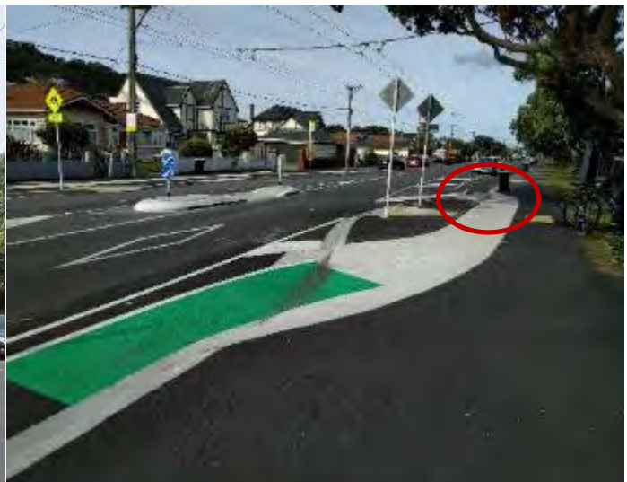
Figure 2-6: Photo showing green coloured cycleway markings provided on departure only. Note also the cycle symbol in advance of the green surfacing blending into the concrete surface
