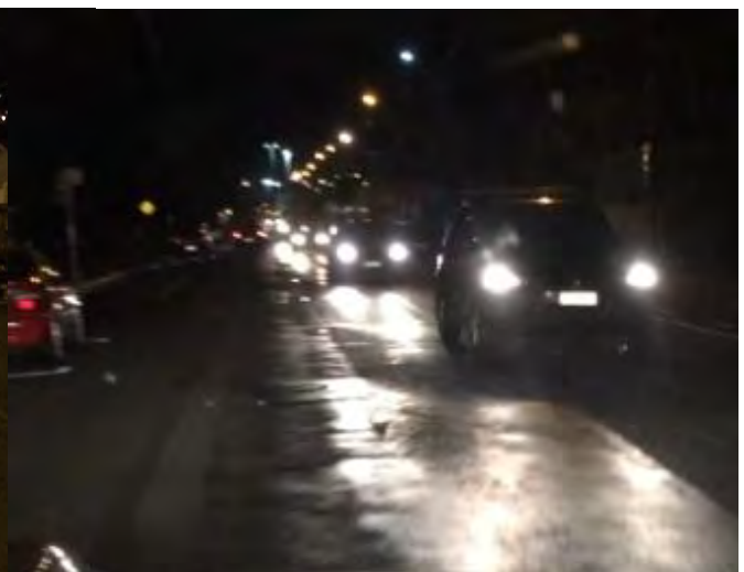
Figure 2-4: Photo showing removal of flush median markings, on a flushed surface, minimises centreline visibility
