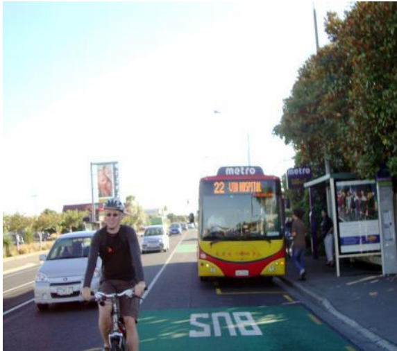
Figure 2-11: Wide transit lane bus stop treatment
