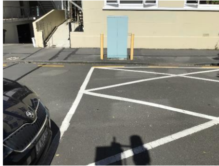
Figure 2-25: Utility kiosk located at proposed crossing point
