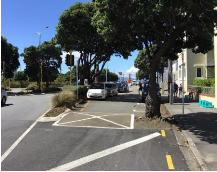
Figure 2-22: Existing speed hump and tree
