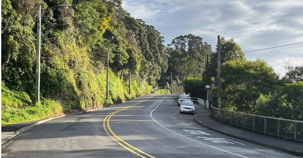
Figure 35: Segment CS-2 Road View
