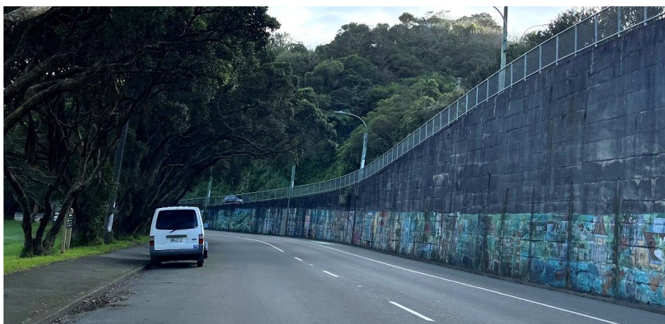
Figure 29: Segment CS-1 Road View
