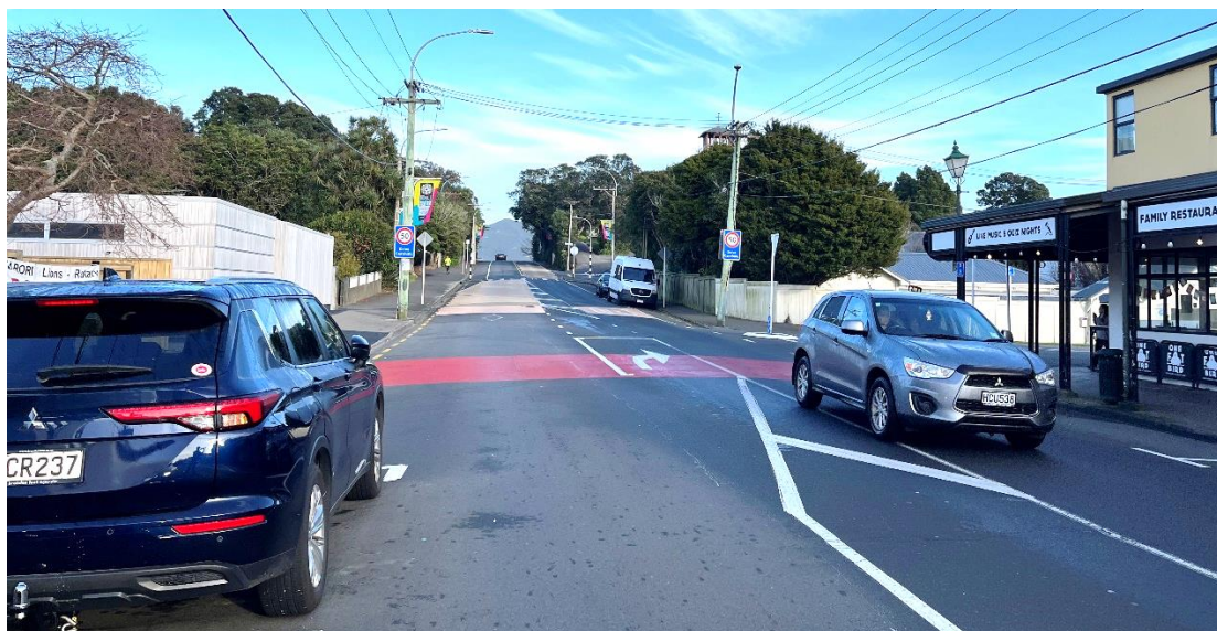
Figure 57: Segment KR-MV-2 Road View
