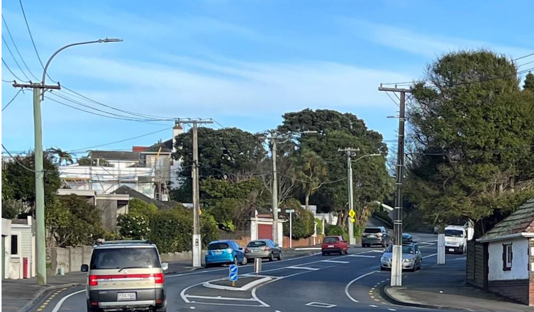
Figure 50: Segment KR-MV-1 Road View
