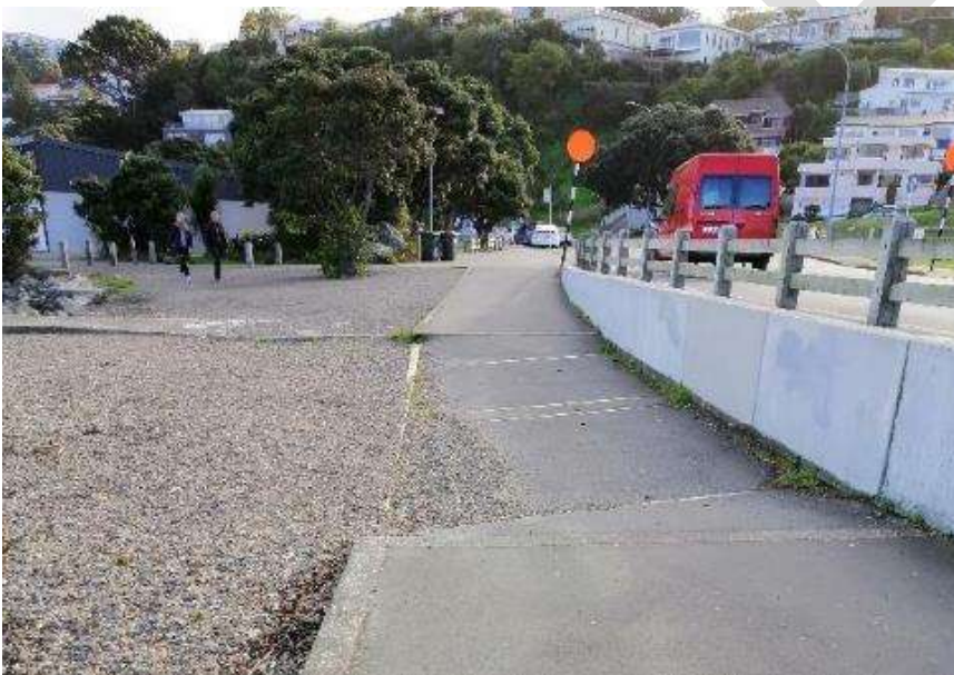
Figure 8: Footpath over patent slip No.2
