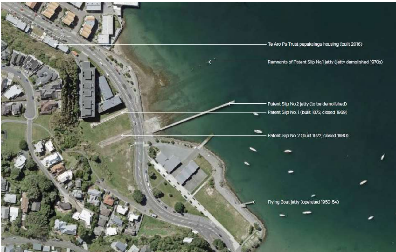
Figure 7: Aerial imagery of patent slip area
