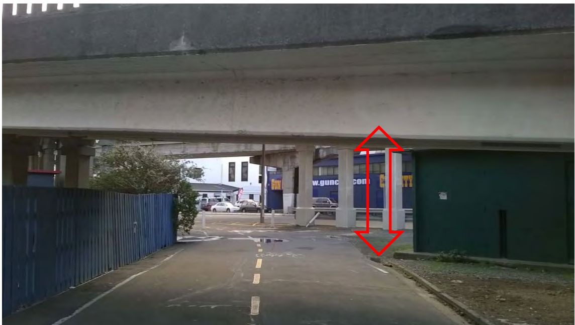
Figure 1 Clearance under Overbridge
