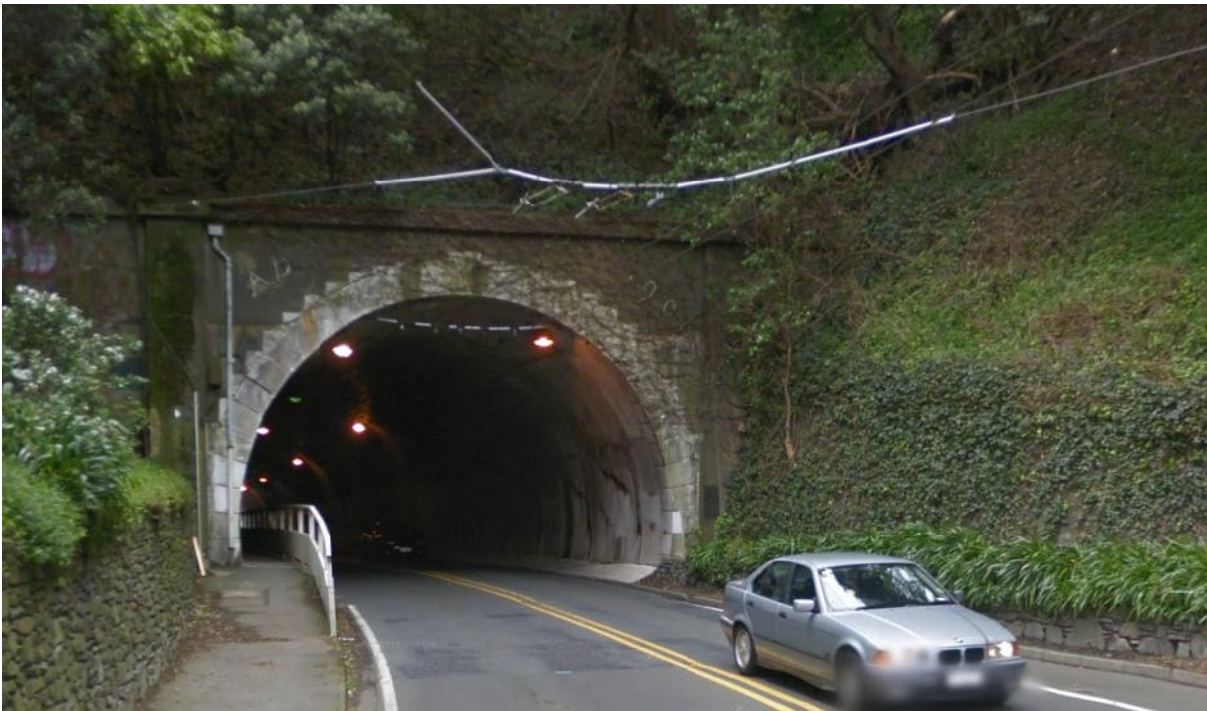
Figure 45 Western end of Seatoun Tunnel 33
