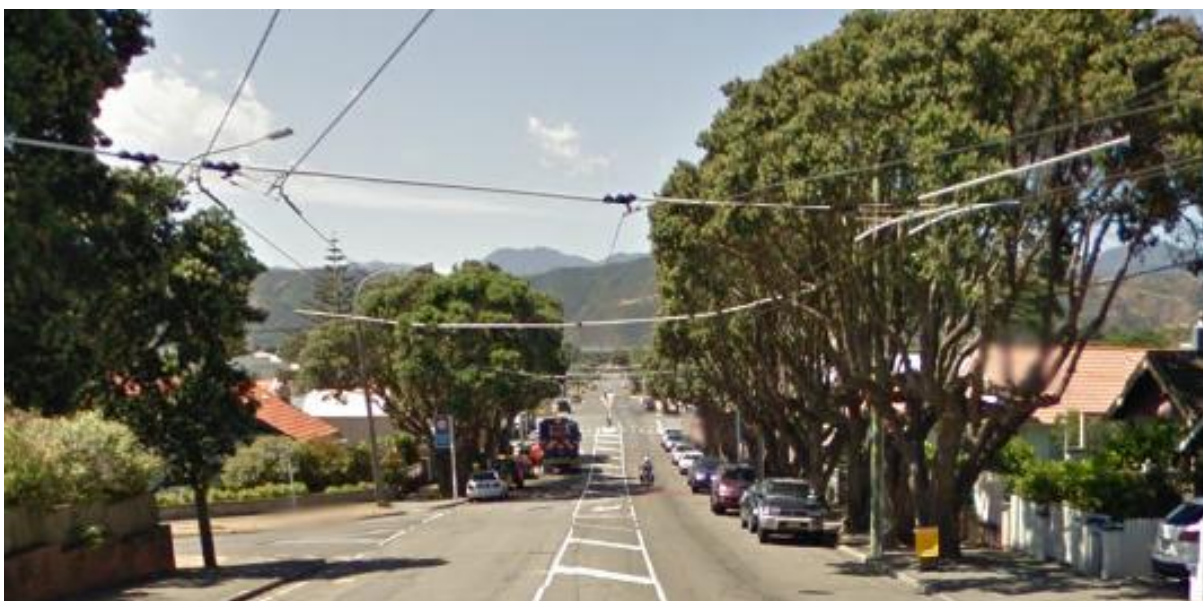
Figure 49 Dundas Street, looking east 36
