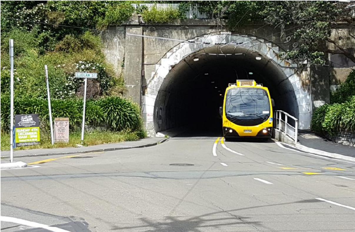
Figure 47 Eastern end of Seatoun Tunnel, looking west
