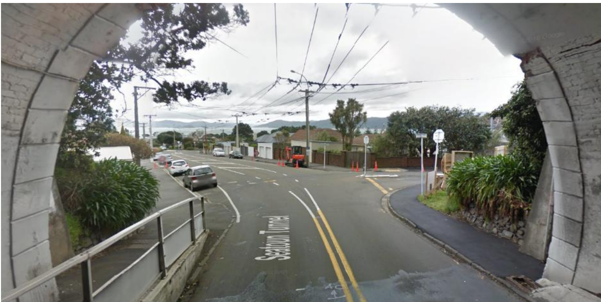
Figure 46 Eastern end of Seatoun Tunnel, looking east 34
