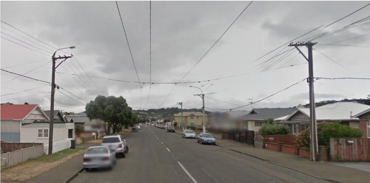
Figure 28 Hobart Street, north of Kedah Street 24
