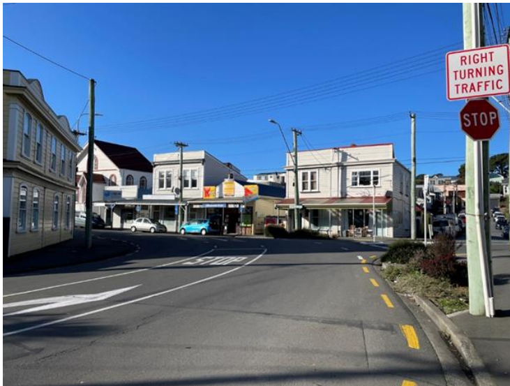
Figure 4-12: Stop applied to right turn bay on Luxford Street into Rintoul Street
