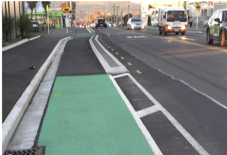
Figure 2.7-1: the leading edge of an island kerb where cycle traffic keeps left and motor traffic keeps right is not to be sign-posted
